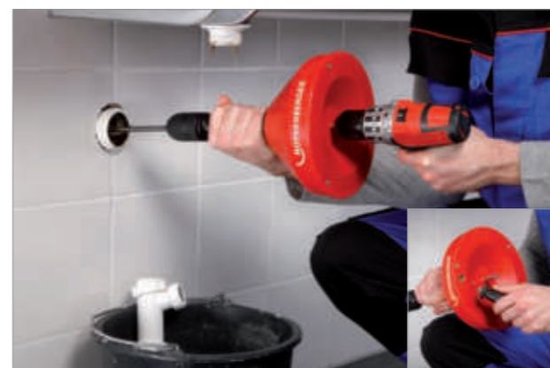
Electrical operation with cordless drill
