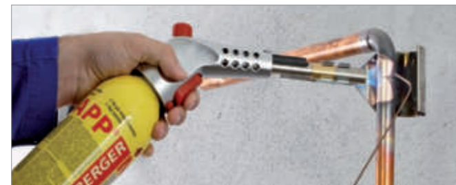
Brazing in gas installation
