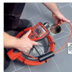
Inspection of floor drains
