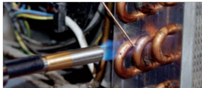
Brazing in aircon and refrigeration
