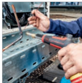
Brazing in aircon and refrigeration
