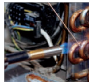
Brazing in aircon and refrigeration
