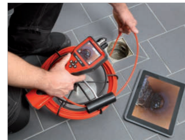
Inspection of basin drains
