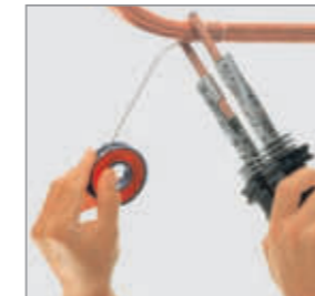
Warming up of the soldering joint without open flame
